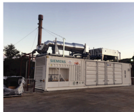
1. Siemens supplied a containerized combined heat and power solution for the ProCaribe liquefied petroleum gas terminal in Puerto Rico. Courtesy: Siemens
