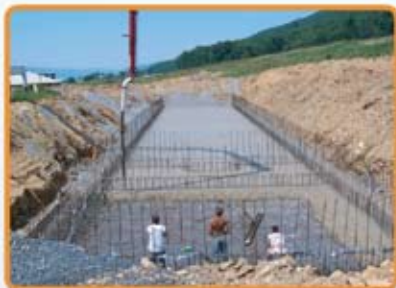
digester under construction
